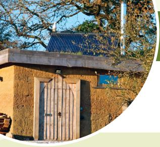
Cob (earthen walled) building for utilities and equipment
